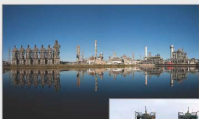
Baytown Olefins Plant
